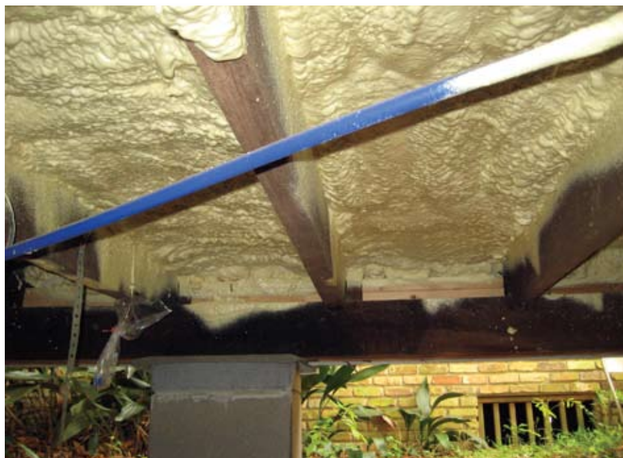
Figure 4b. Example of closed cell spray foam.
