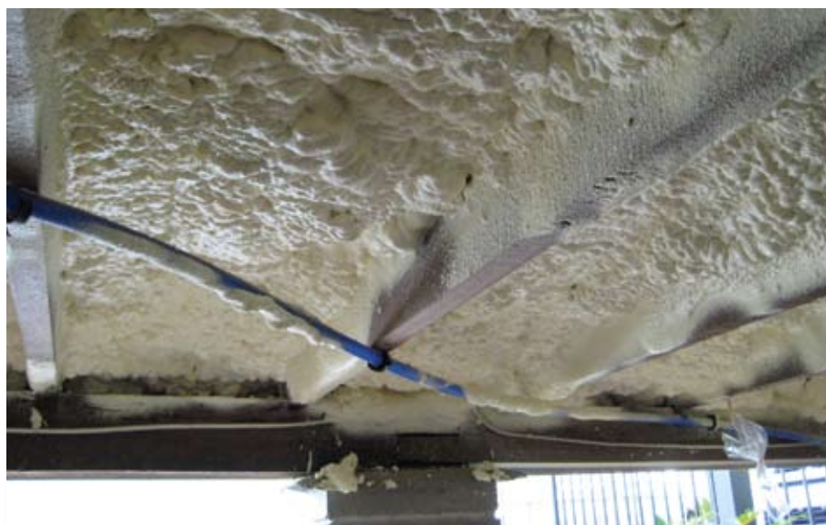
Figure 4c. Example of open cell spray foam.
