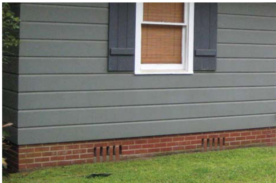
Figure 2. Example of a wall-vented crawl space.
