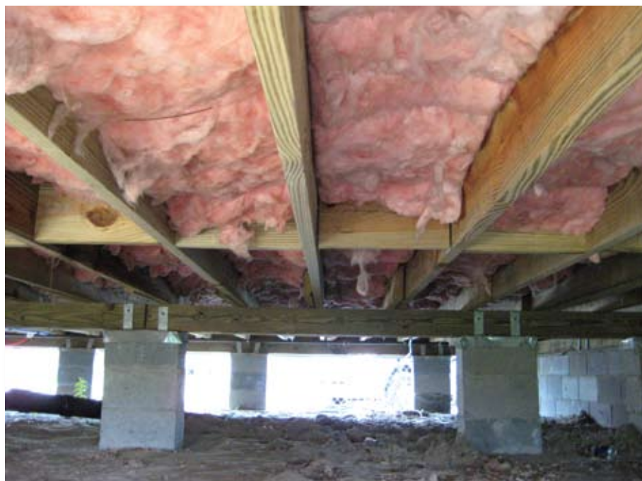
Figure 4d. Example of typical fiberglass batt insulation.
