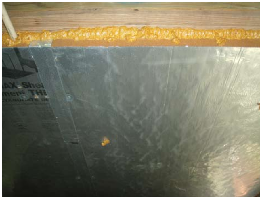
Figure 4a. Example of rigid, foil-faced polyisocyanurate foam.
