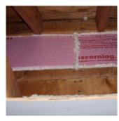
**Figure 10.** When researchers pulled back the porch ceiling, they found the wall board was missing so nothing was covering the insulation on this exterior wall. An air barrier of rigid foam board was put in place with spray foam (Image: Moriarta 2008).
