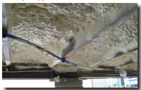
Figure 4c. Example of open cell spray foam.
