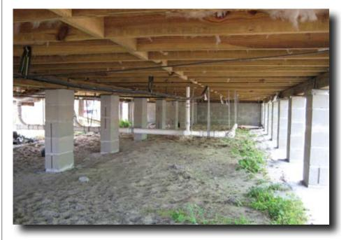
Figure 1. Example of an open crawl space.
