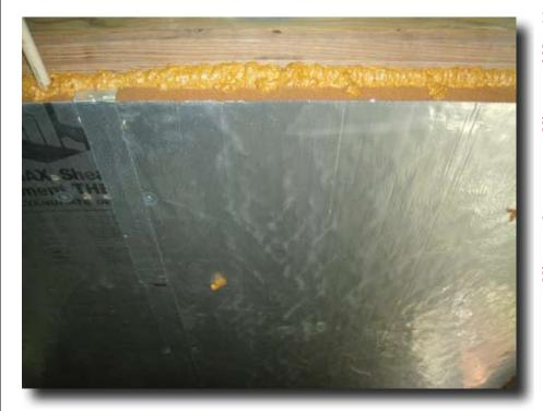
Figure 4a. Example of rigid, foil-faced polyisocyanurate foam.
