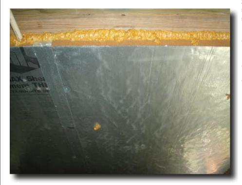
Figure 4a. Example of rigid, foil-faced polyisocyanurate foam.
