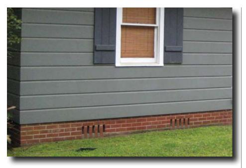
Figure 2. Example of a wall-vented crawl space.
