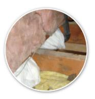
Figure 6. Air seal floor joist cavities under kneewalls by filling cavities with fiberglass batts that are rolled and stuffed in plastic bags (as shown here) or use rigid foam, Oriented Strand Board (OSB), or other air barrier board cut to fit and sealed at the edges with caulk.
