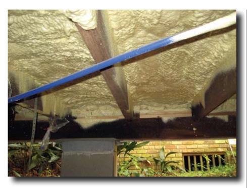
Figure 4b. Example of closed cell spray foam.
