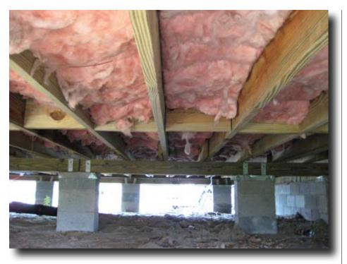
Figure 4d. Example of typical fiberglass batt insulation.
