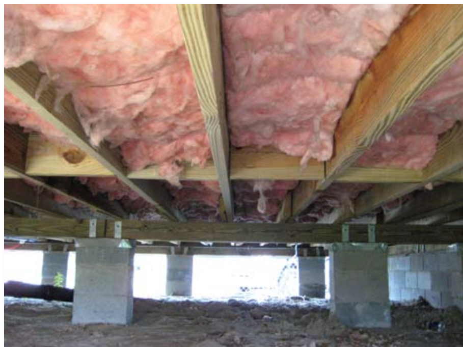
Figure 4d. Example of typical fiberglass batt insulation.
