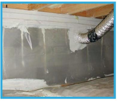
There is no polyethylene sheeting installed in the crawlspace.
