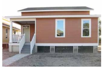
Photograph 7: Elevated and Open Crawlspace—Open pier construction and a trellis couple the crawlspace to the exterior.
