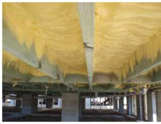
**Photograph 6: Spray Foam Between Joists**—Floor framing is not completely encased with spray foam in this application. Works only where the crawlspace is open to the outside.
