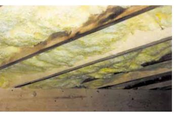
**Photograph 1: Icky Crawlspace**—Note the condensation on the underside of the fiberglass insulation and the rot at the exposed portions of the crawlspace floor joists.
