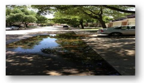
were noted on many streets where either the underlying subgrade contracted causing a dip in the gutter line or the fat clays expanded in an area causing the pavement to heave. Again, the City of Bellaire topographically, is very flat, sloping only about 5 ft. over 10,000 feet or a little over half an inch in 100 feet. Consequently, our street and gutter system is flat as well. So, any adverse movement in the gutter can create street ponding.
