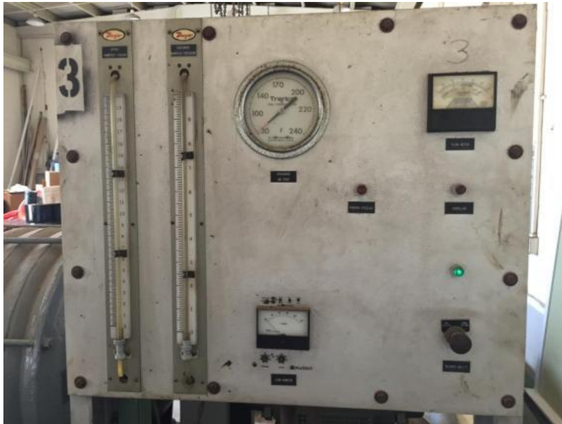
Antiquated blower control panel – Gauges not functional
