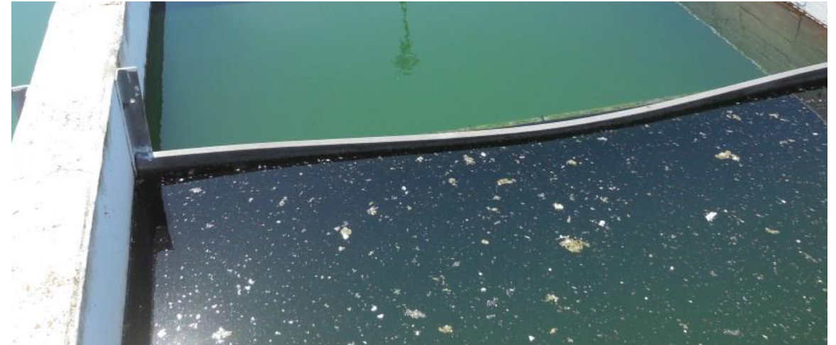
Chlorine Contact Chamber – broken baffles – infiltration issues – below 100yr floodplain
