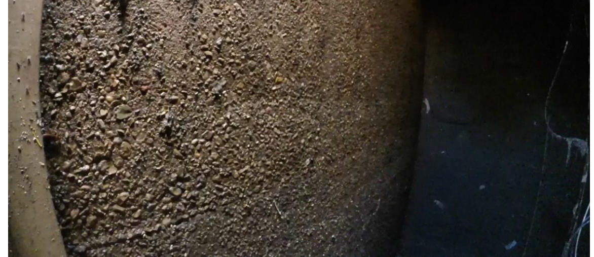
Corrosion of concrete walls
