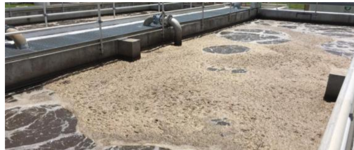
Foam indicates fine bubble diffusers may be clogged
