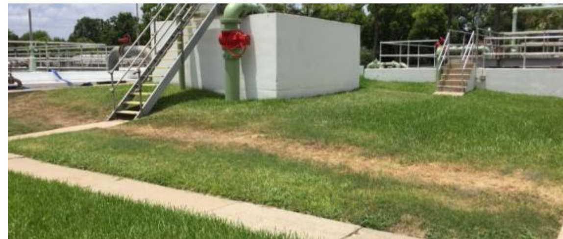
Grass not growing is area above piping—indicator of piping leaks
