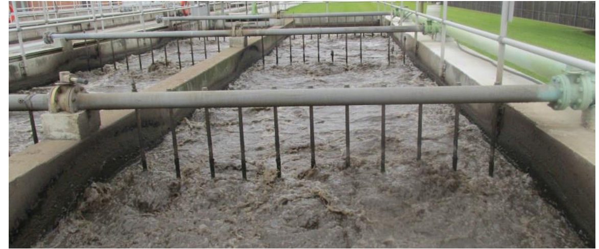
Pre-aeration basin – coarse bubble diffuser
