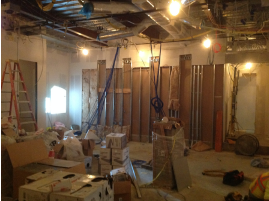
PD dispatch room picture taken Sept 4 Removed sheetrock for all video wall issues RFI 212, 216 & 221
