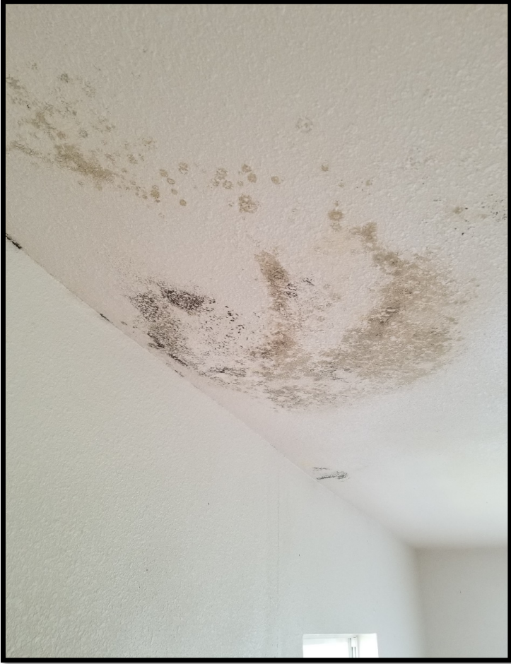
Roof Leak
